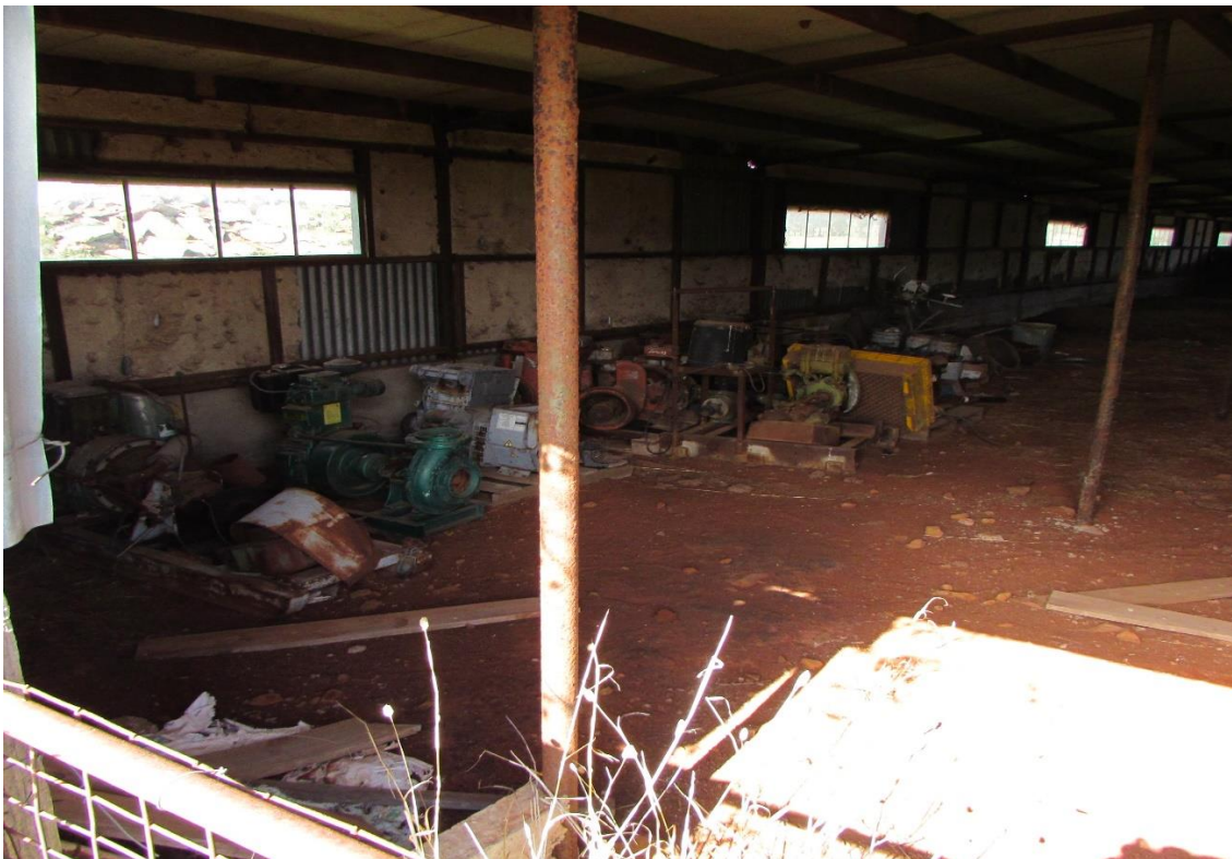
Figure 6.5-Engines stored in the livestock shed.
