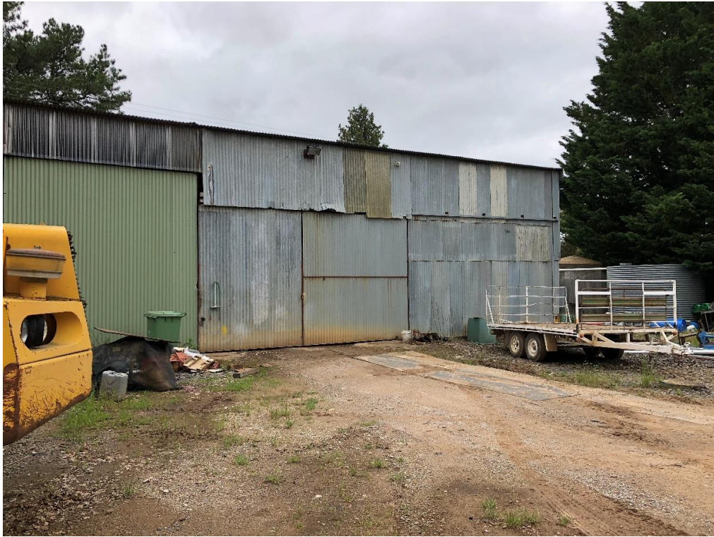
Figure 6.9: Workshop shed with concrete slab on ground and gravel stabilised access.
