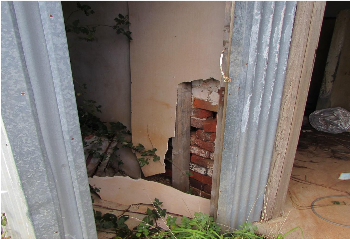
Figure 6.4- Fibre-cement sheeting observed in structure at the Subject Site.
