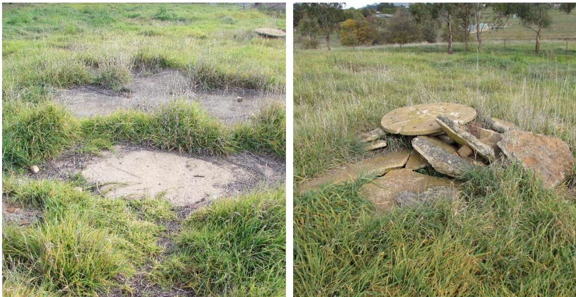
Figure 6.1 – Concrete pad and broken concrete south of existing dwelling.
